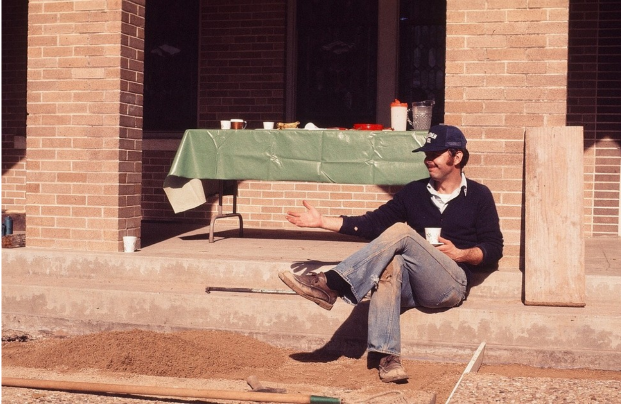
2/76 John Camden doing an excellent job of supervising the leveling of the church courtyard
