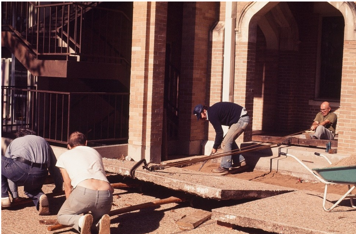
2/76 John Towery, Mel Oakes, John Camden, and Rizer Everett working on leveling the courtyard which was sinking
